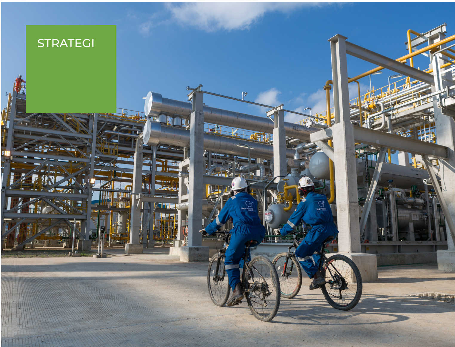
Central Processing Plant, Block A, Aceh Timur, Indonesia
